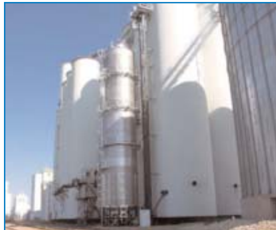
The new grain dryers that have been installed at the Cherokee location (left photo) and the Marcus location (right photo) are both 4,000 bushel per hour systems and will greatly enhance grain drying speed and capabilities for our customers this fall and for many seasons into the future.
