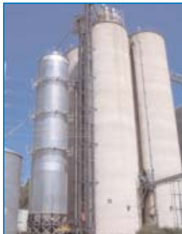
The new grain dryers that have been installed at the Cherokee location (left photo) and the Marcus location (right photo) are both 4,000 bushel per hour systems and will greatly enhance grain drying speed and capabilities for our customers this fall and for many seasons into the future.
