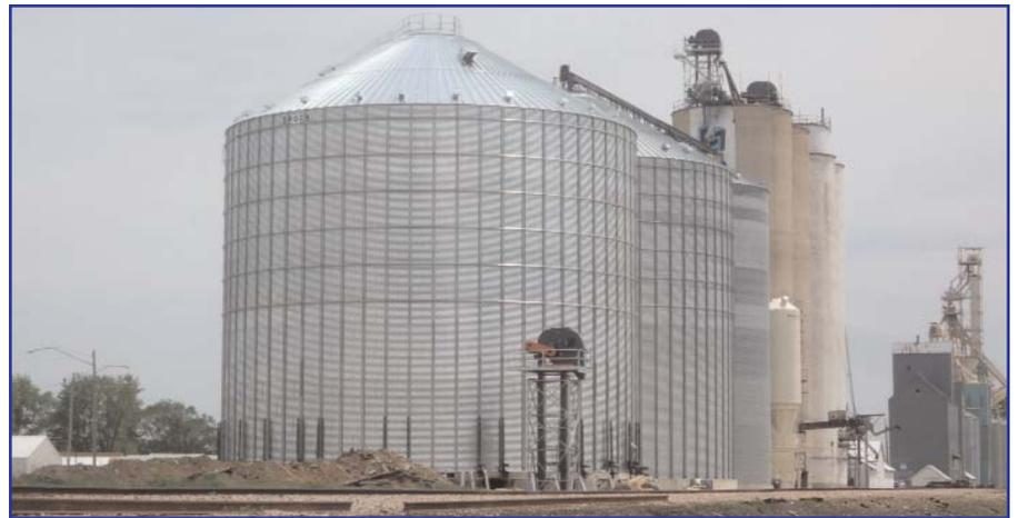
*The new 500,000 storage bin at Alta featured in this photo is one of several exciting construction projects for 2011 in FCA's on-going grain receiving, drying and storage upgrades. Also included in this project is a 13,500 bushel per hour covered dump pit and 4,700 bushel per hour grain dryer. A new office, scale and warehouse complex will also be built this summer.*
