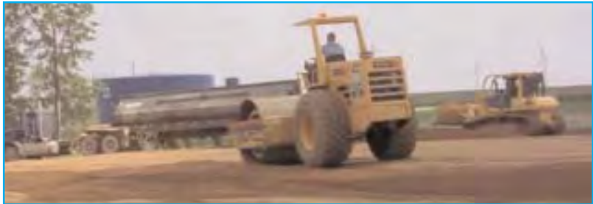
Excavation work was continuing on the new bulk fertilizer plant at the FCA Aurelia location as tons of dirt were being moved and sand was being hauled in to prepare the storage facility foundation.
