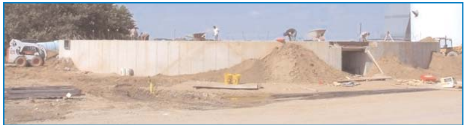
A New 500,000 Bushel Bin Takes Shape At Marcus
